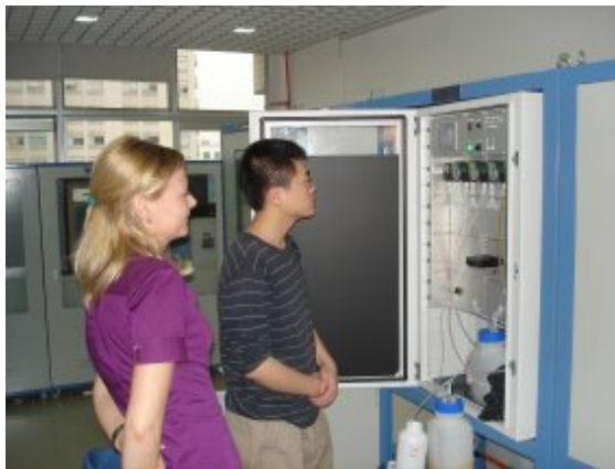
Fig. 6: Installation in Shenzhen/China.
