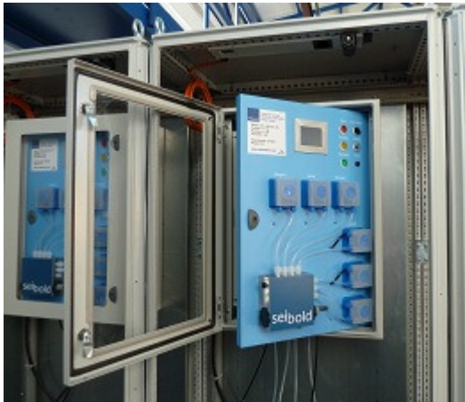
Installation: Drinking Water Plant
